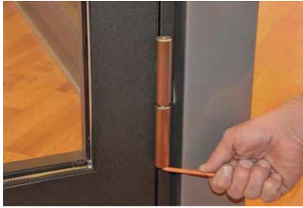
Drive a 5mm Allen key through the hollow lock nut and move door leaf up or down by turning the hinge bolt with the key. After adjusting the height fix bolt with the lock nut.
