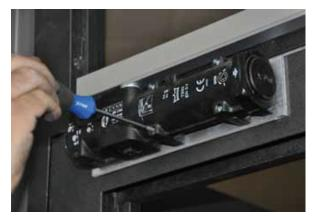
Doors are fitted with Dorma TS 93 door closers see specific manufacturer's instructions for closer adjustments.
