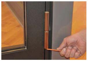
Drive a 5mm Allen key through the hollow lock nut and move door leaf up or down by turning the hinge bolt with the key. After adjusting the height fix bolt with the lock nut.
